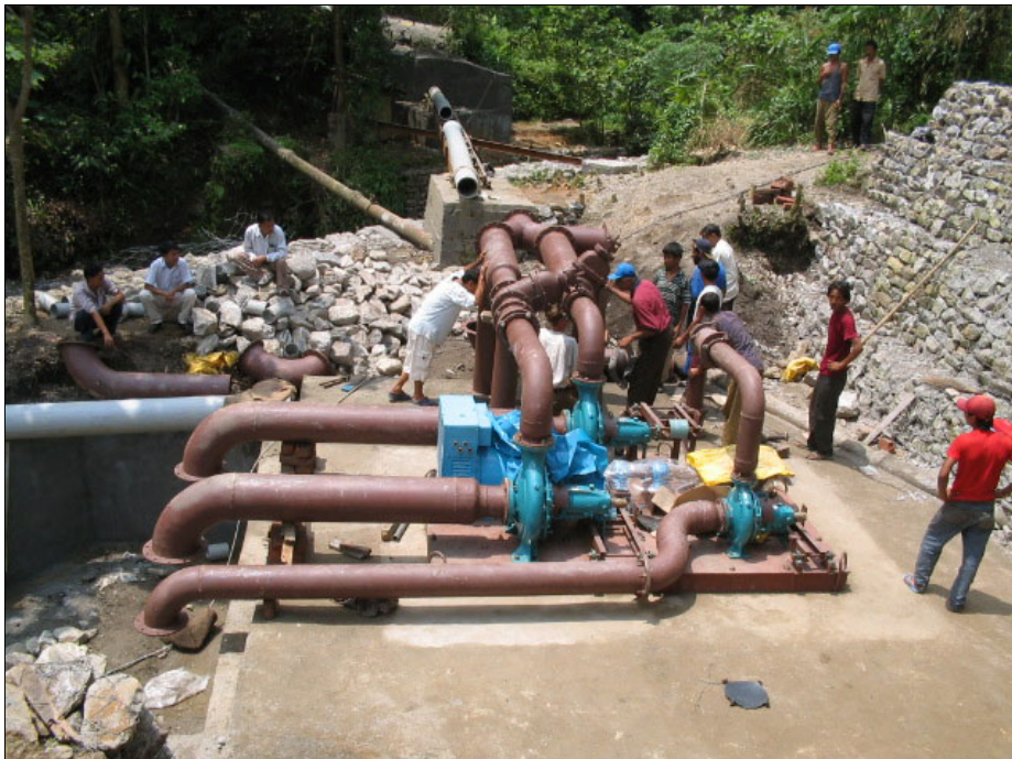
Figure B6.24 , Installation of the Manifold Lines and Draft Tubes
