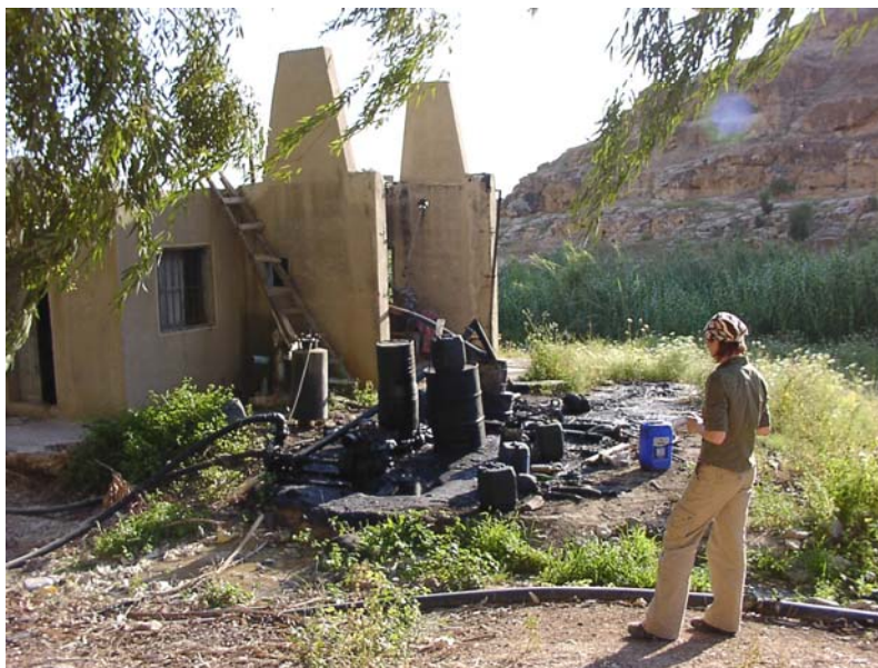
Fig. 8.6: Leaking oil pump in the test area causing a significant point hazard.
