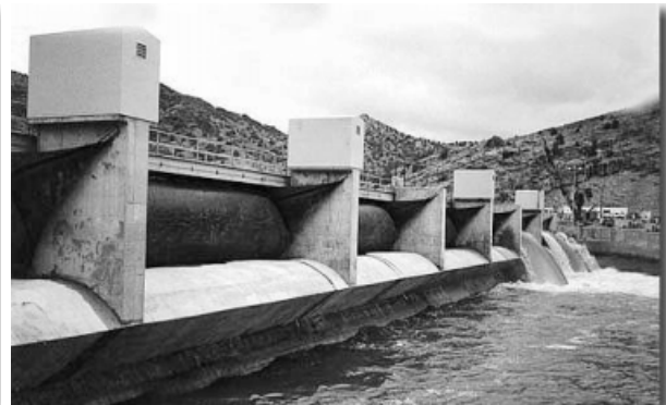
Hakone 2 Hydroelectric Power Production, Japan (7 x 15,00 x 3,35 m)
