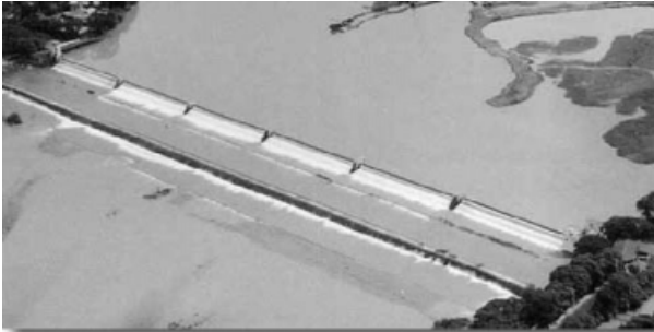
Angat After Bay Regulator Dam, Philippinen (6 x 13,17m x 2,50 m)
