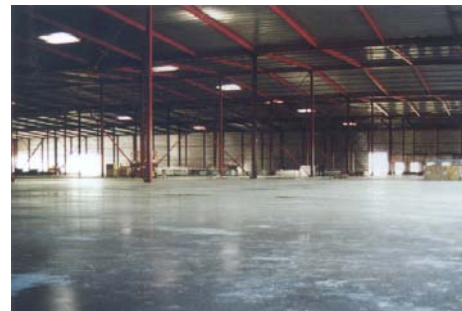
Fig. 11: Industrial floor on piles in steel fibre reinforced concrete.
