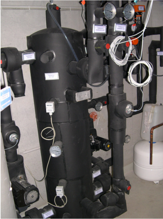
Abb. 16: Solar-Pufferspeicher
