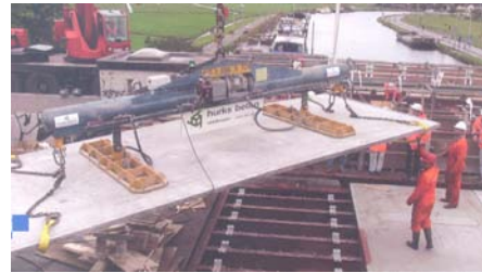
Fig. 21: Bridge deck of ultra high strength fibre concrete as a substitute for a deck of tropical wood.
