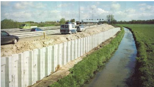
Fig. 17: Concrete sheet piles for soil retainment.
