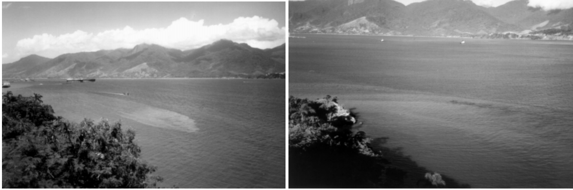
Fig. 4: Aerial view of an outfall, discharging in the São Sebastião channel at two different time-steps, showing completely different dispersion patterns (Lamparelli, 2003).
