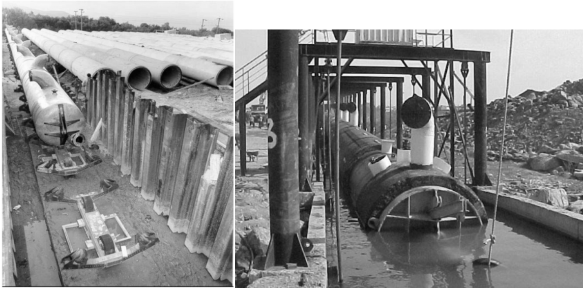
Fig. 18: Pictures of multiport diffusers during construction (Bonnasabla.com)
