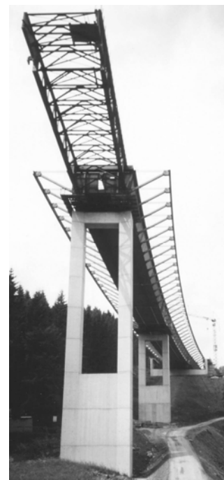
Bridge (Sessles Valley)
