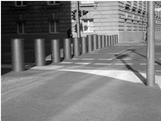
Additional safety measures: sliding bollards
