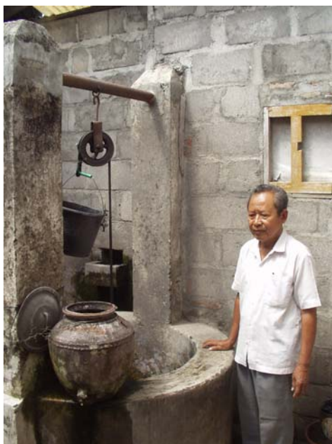
Figure 4.41: A dug well in Prambanan has a serious groundwater fluctuation between the dry and rainy seasons (Photo: Widodo, July 2005)
