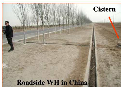
Figure 5.14: Catching runoff from highway and storing the water for other purposes, a case in China
