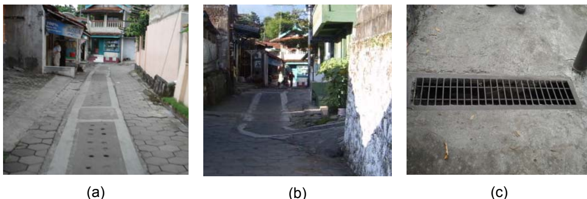
Figure 5.10: Patterns of drainage channels: (a) along the street, (b) bended channel, and (c) crossing the street
