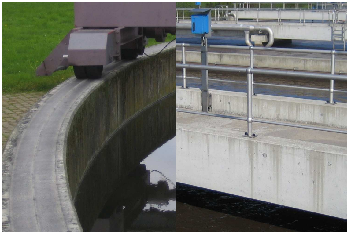
FIGURE 152: CONCRETE STRUCTURES ON STPS IN GERMANY
