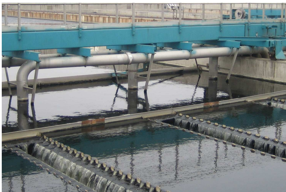
FIGURE 101: WEIR EDGES AND BRIDGE IN CHINA
