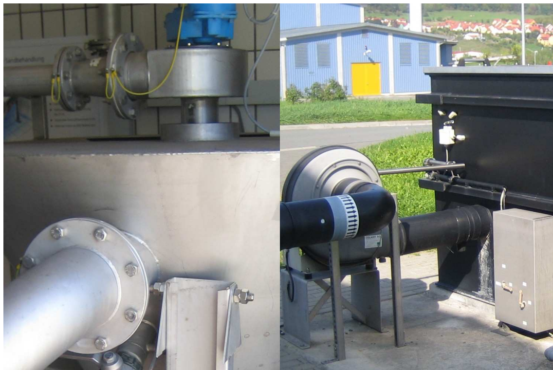
FIGURE 163: CORROSION RESISTANT MATERIAL OF MACHINERY EQUIPMENT IN GERMANY
