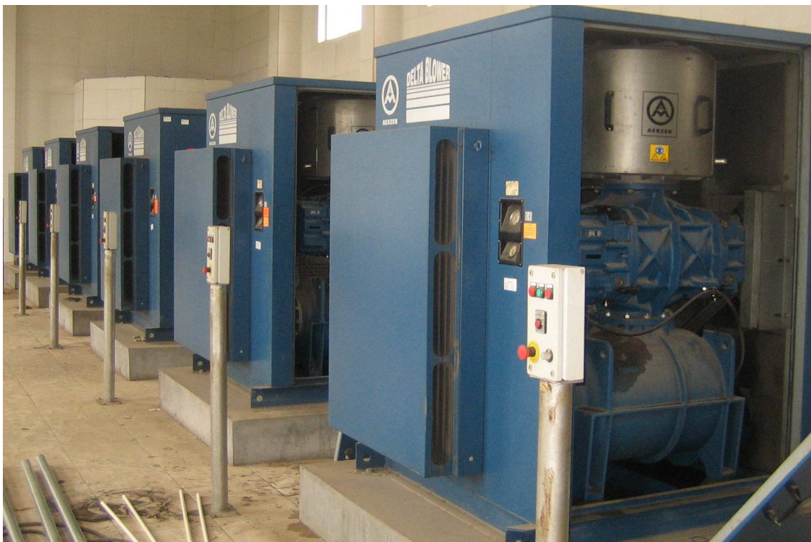
FIGURE 112: IMPORTED ROTARY PISTON VALVE COMPRESSORS IN CHINA
