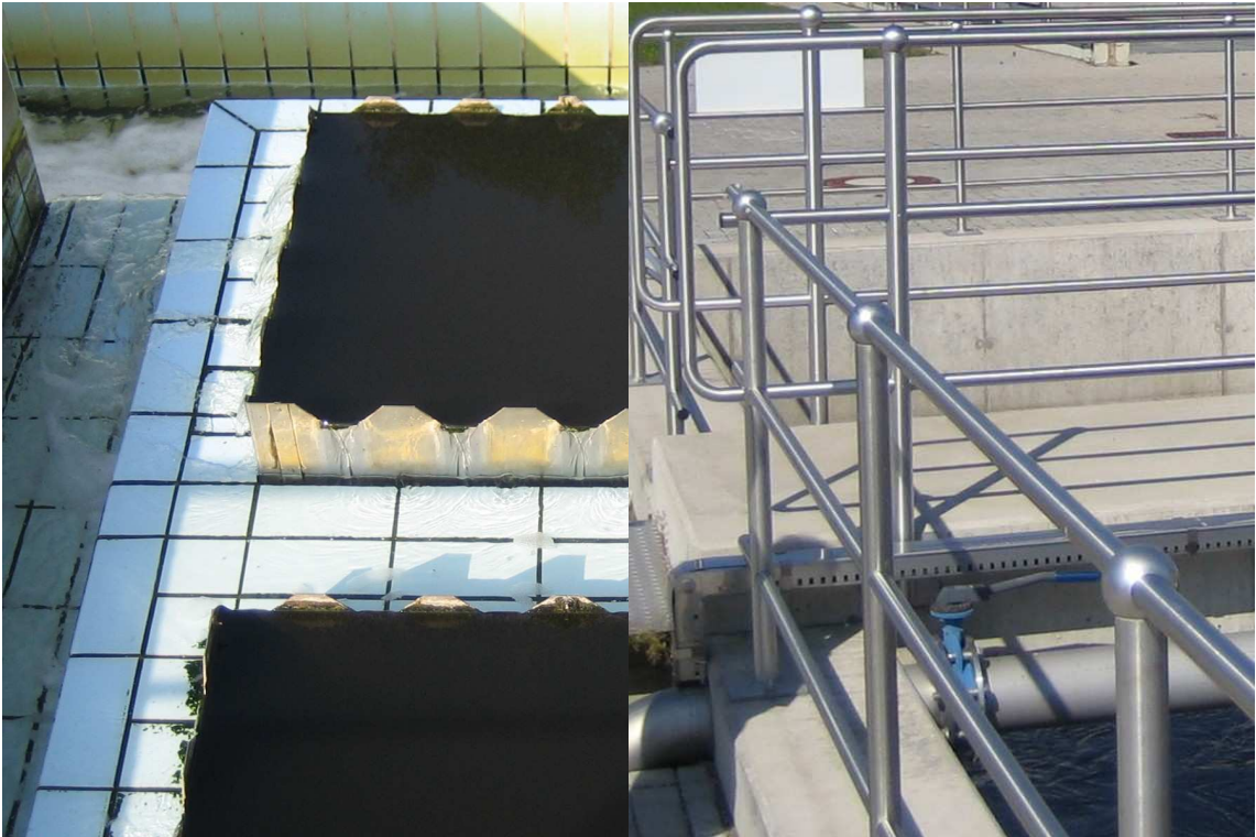
FIGURE 153: WEIR EDGES AND HANDRAILS ON STPS IN GERMANY
