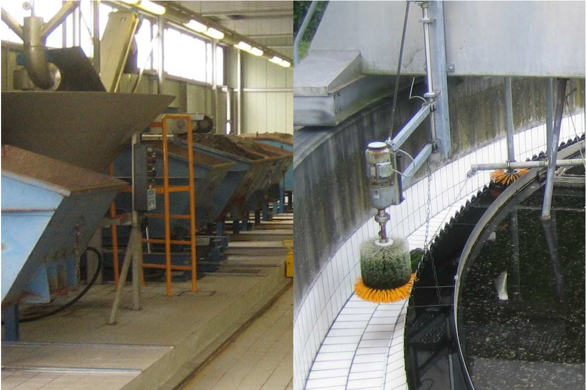
FIGURE 154: CLEANLINESS OF PLANT EQUIPMENT IN GERMANY
