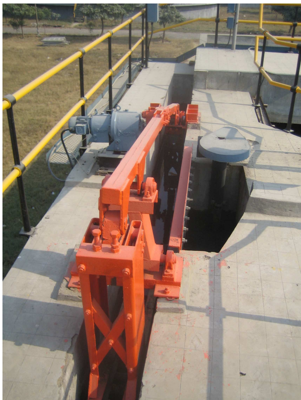
FIGURE 57: WELL COATED GRIT REMOVAL SYSTEM IN INDIA
