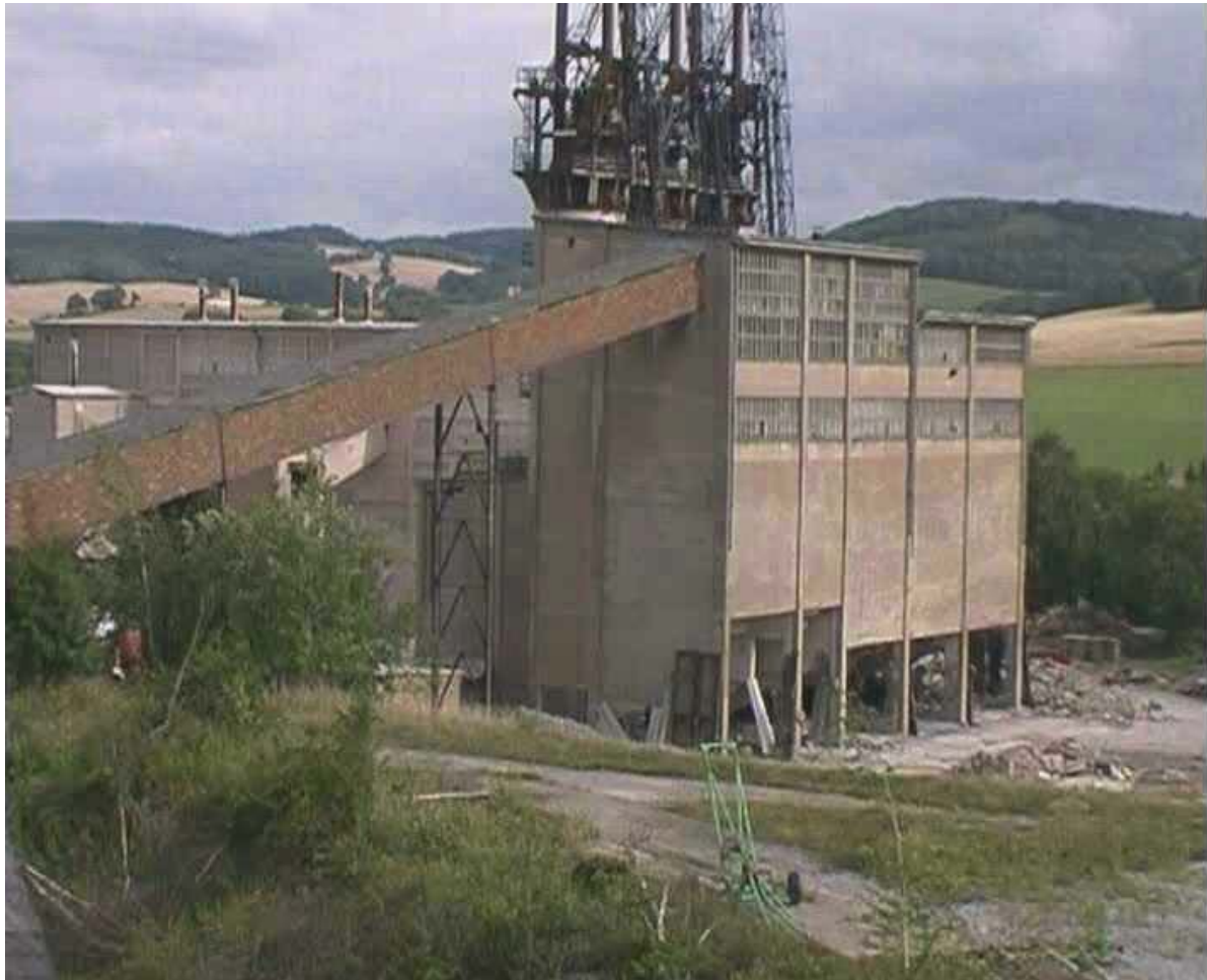
Figure 1: Investigated structure, Silo building at the lime works in Borna
