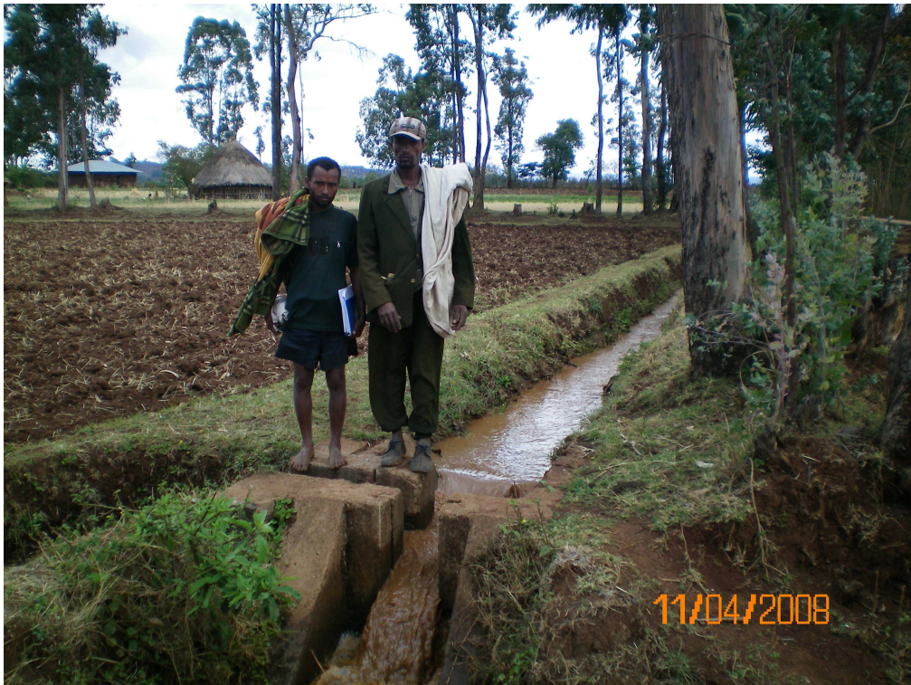
Figure 31 A drop structure combined with a turnout along the tertiary canal
