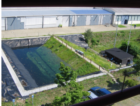
Figure 3.1: View from top on the full-scale dike model at the Federal Waterways Engineering and Research Institute Karlsruhe, Germany, during the flooding experiment.
