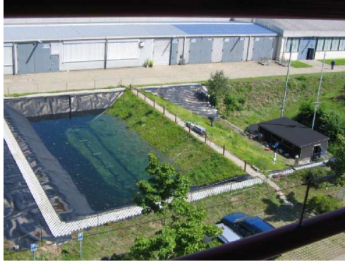
Figure 3.1: View from top on the full-scale dike model at the Federal Waterways and Research Institute Karlsruhe, Germany, during the flooding experiment.
