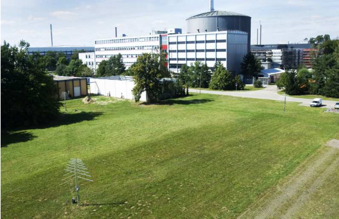
Figure 3.2: Part of the antenna cluster D30. The triangular structure of the antenna positions and the north-south & east-west polarisation are clearly visible.
