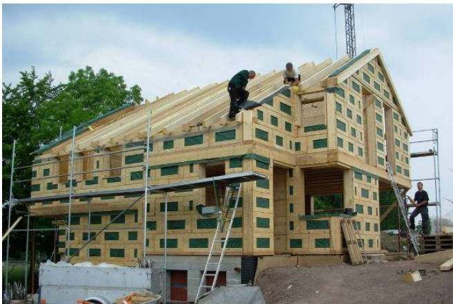
Fig. 1 Building made of Prefabricated Timber Wall Elements
