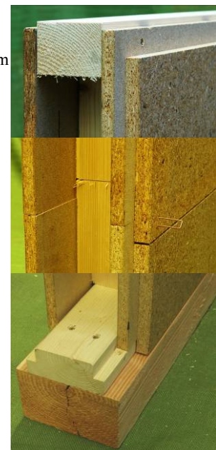
Fig. 4 Details of Prefabricated Timber Wall Element System
