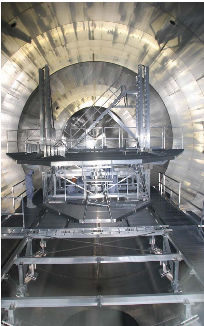
Figure 2.7: The inside of the Main Spectrometer vessel. The photo shows the inside of the Main Spectrometer vessel during construction of the scaffolding that is needed for mounting of the inner wire electrodes.
