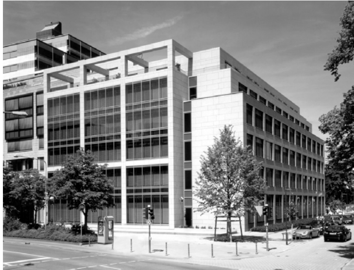
Figure 1. The south-elevation of the new KfW building
