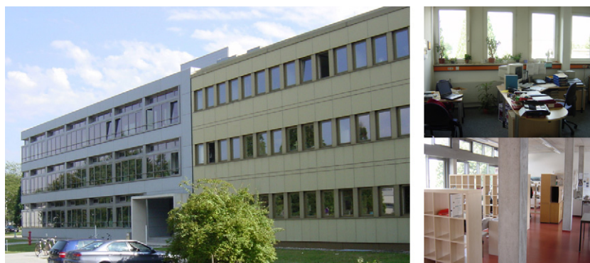
Fig. 1. View of the whole building from the north (right: existing part, left: new extension) and views of two different offices (top: existing part, bottom: new extension).
