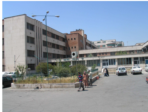
Figure 4-6: Tebie Kudakan Hospital
