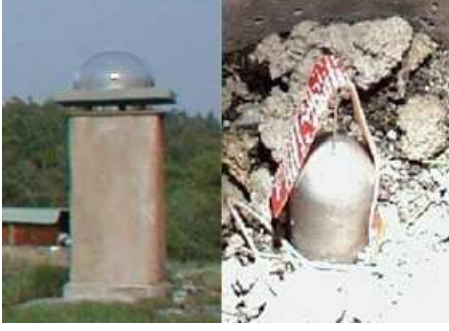
Figure 1. IGS-reference point (right) in the IGS-monument (left).
