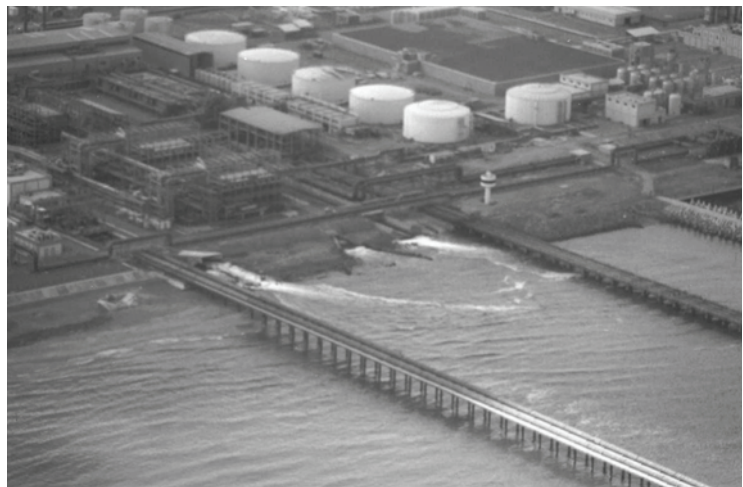
Fig. 1: Al Ghubrah desalination plant (largest in Oman, production capacity 191,000 m 3 /d): Brine waste discharge through an open channel at the beach into the Gulf of Oman (photo: H.H. Al-Barwani)
