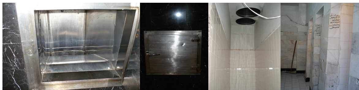
Figure 5-46: Dirty washing collection (Iran)
