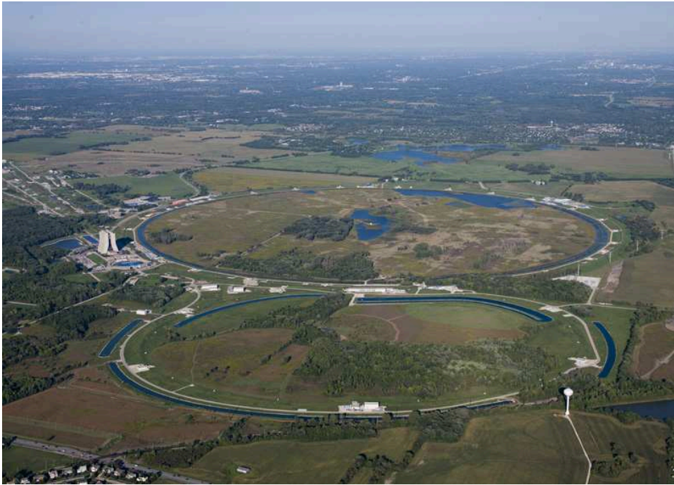
Figure 3.1: The Tevatron from a bird's eye view. The Tevatron is located in the center of the picture under the upper of the two visible rings.
