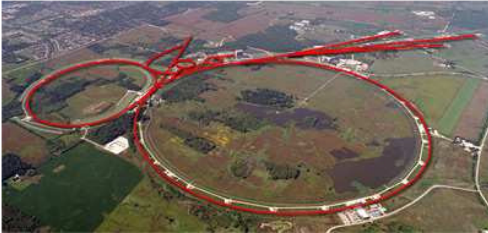
Figure 2.1: Aerial view of the accelerator complex at Fermilab. Tevatron itself is of course underground. However, the maintenance road in the middle of the picture, nicely indicates its course. Tevatron hosts two multipurpose detectors: CDF II and D\bar{O} .
