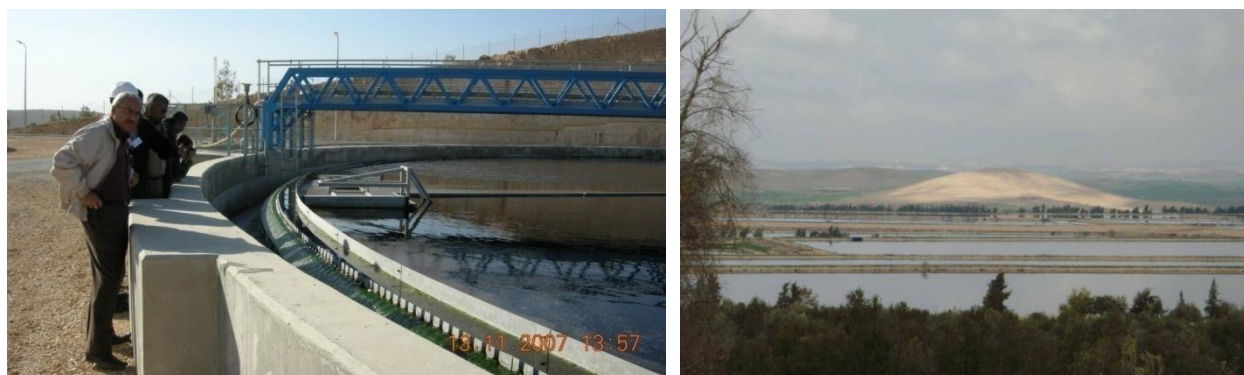
Figure 3-1: As'samra waste stabilization pond, the new WWTP to the right and old to the left (Pictures taken on Nov, 2007).
