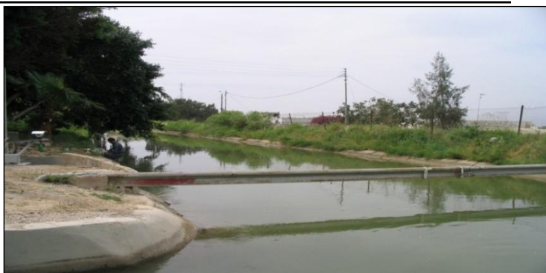
Figure 2-3: King Abdullah Canal (KAC) in the north of JV.
