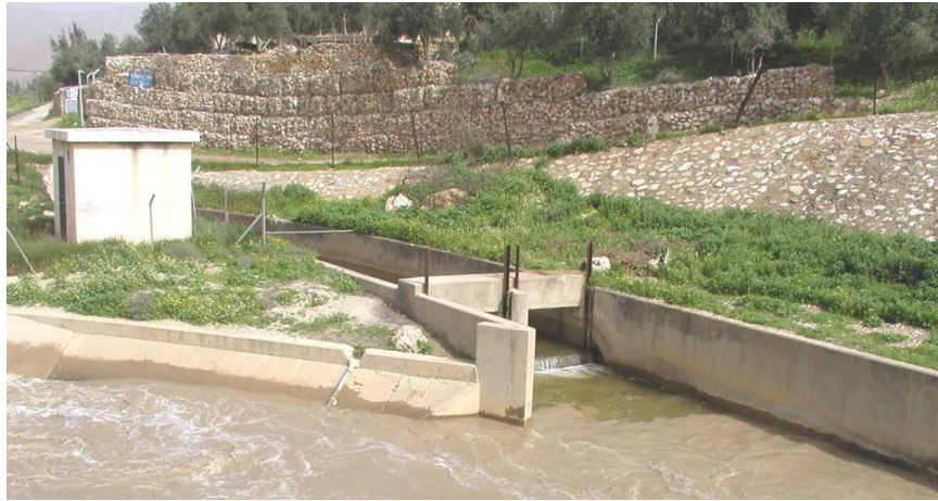
Figure 2-5: Mixing point for treated wastewater from King Talal Reservoir (right) and fresh surface water from the Yarmuk river deviated in the King Abdullah Canal (left).
