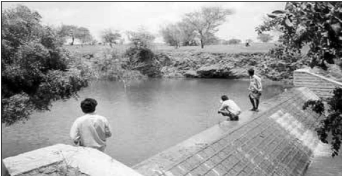
Figure 4.12: Check dam in the catchment (Wani et al., 2003)
