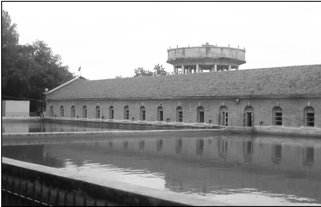
Figure 2.27: Raw water treatment facility downstream of Osman Sagar reservoir
