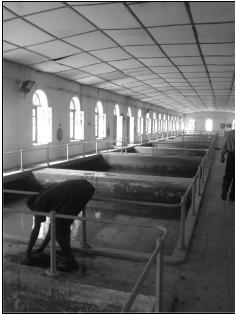
Figure 2.29: Rapid Gravity Filters at raw water treatment plant
