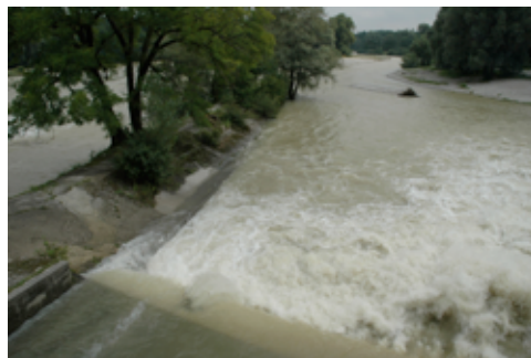
Fig. 2: Isar River flooding [Photo Torben Dam]
