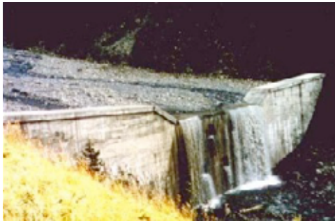
Fig.3: Massive concrete weir [Photo: Henn 1998: 4]
