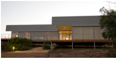
Fig. 13: The Hollingworth House – Point Henry, WA (fire shutters down at dusk) [Photograph by Andrew Halsall 2008]
