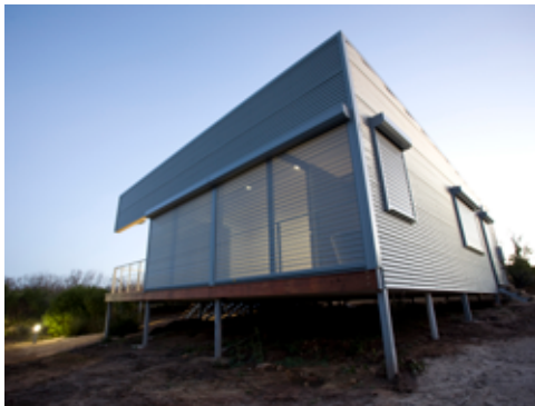
Fig. 14: The Hollingworth House – with the perforated fire shutters down at dusk. [Photograph by Andrew Halsall 2008]
