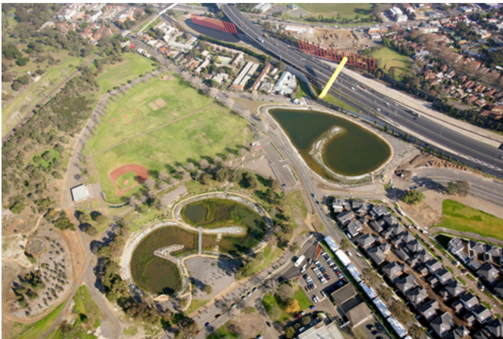
Fig. 3: Aerial view of Royal Park Wetlands by Rush Wright Associates
