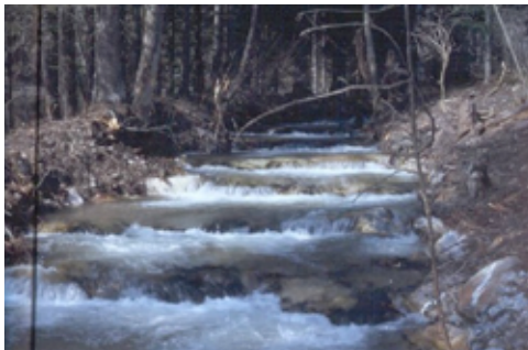
Fig.4: Near-natural Pendelrampe ('weaving chute') instead of a concrete weir [Photo: Grober]
