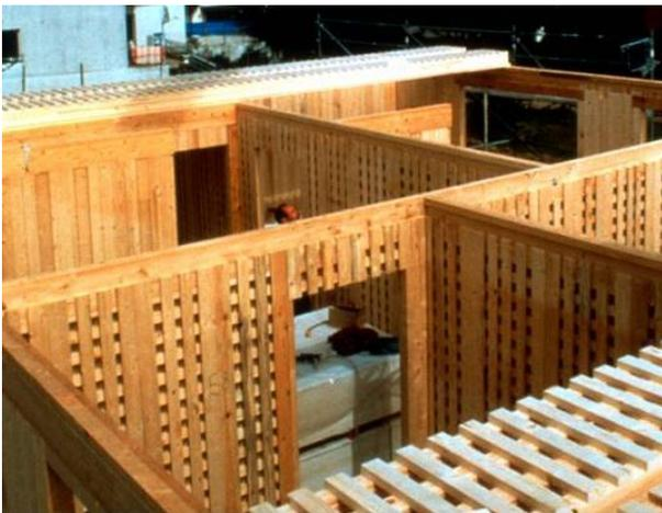
**Figure 2:** Building made of X-lam massive panels
