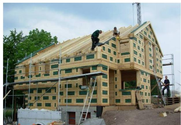
**Figure 4:** Building made of prefabricated timber wall elements
