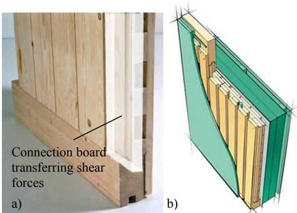
**Figure 1:** a) Close-up view of the bottom of a single X-lam massive panel, b) Panel with inner finish plus installation and outer insulation
