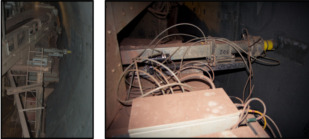
Figure 2.9.: Pneumatic hammer source applied at the tubing segment. These picture have been taken during a seismic survey conducted in the Neuer Schlüchterner Tunnel close to Fulda, Germany.
