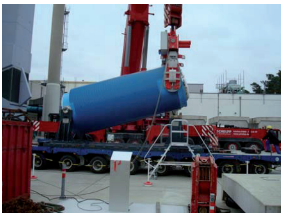
Fig. 7: Handling of the CASTOR cask outside VEK
