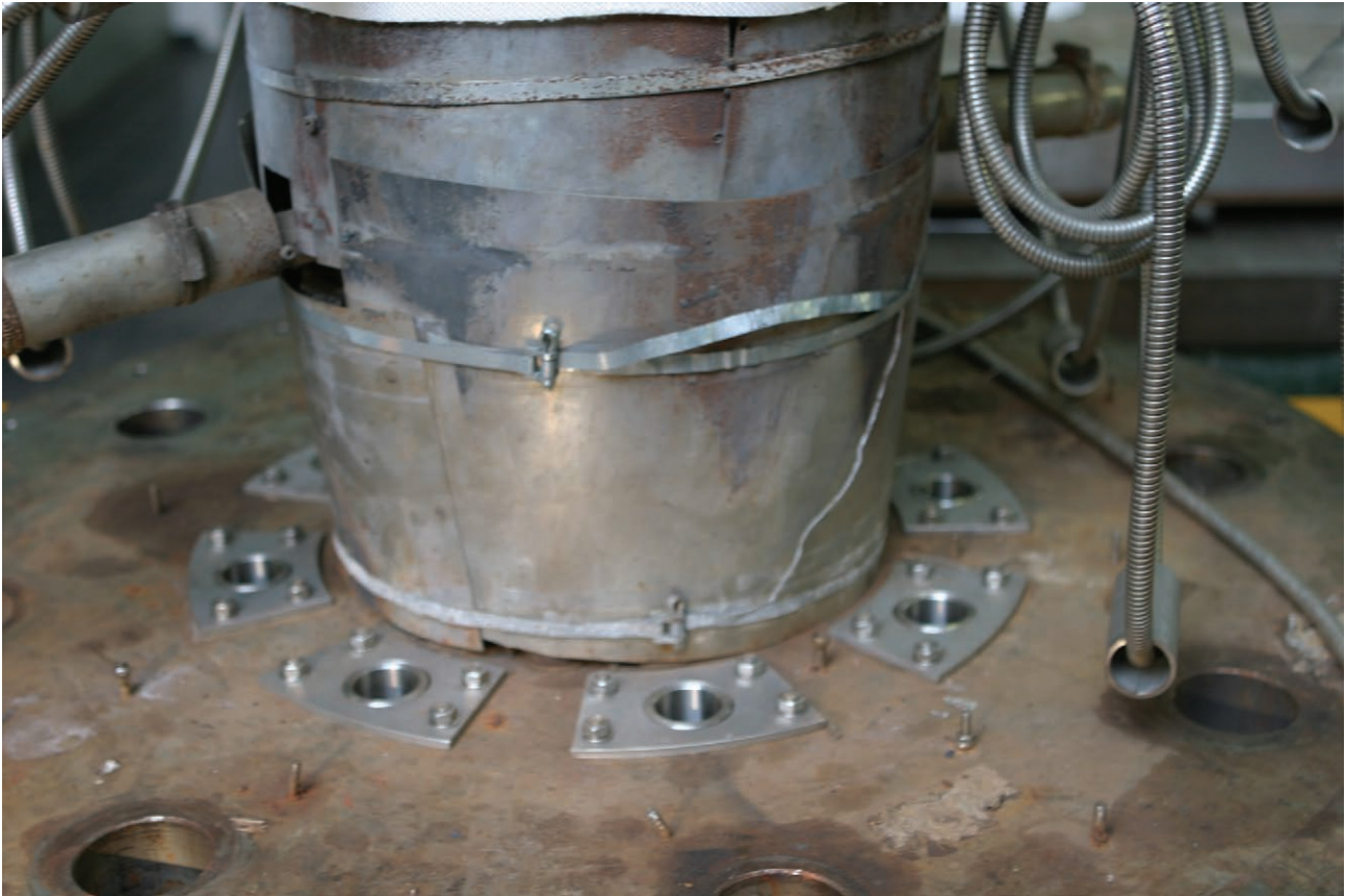
Fig. 3-7. Top view of the cavity top plate with exit holes leading into subcompartment 2
