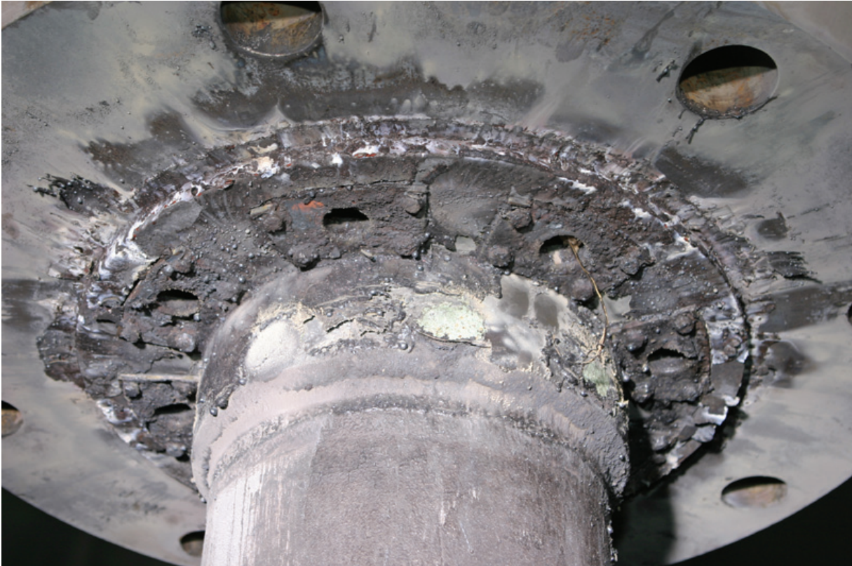
Fig. 4-17. KH01: View at pit exit B leading into subcompartment 2
