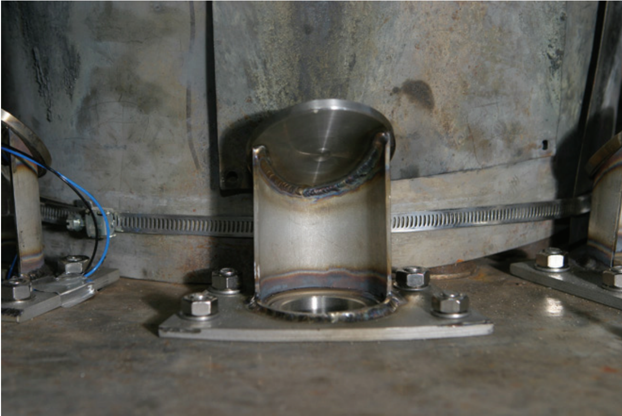
Fig. 4-109. KH04: Exit of path to refueling room (subcompartment 2)
