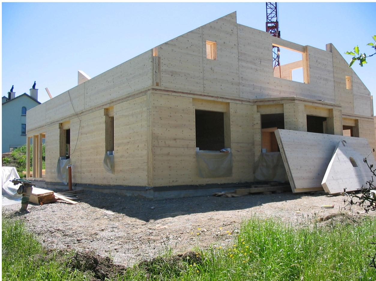
Fig. 3 Massive timber building made using CLT panels
