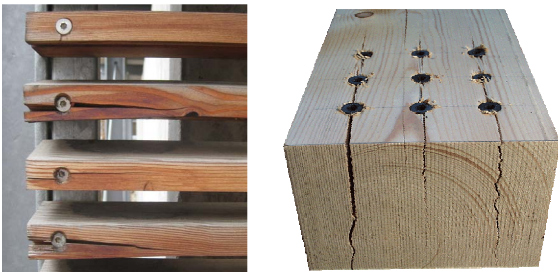
Fig. 1: Typical splitting failure caused by the insertion of self-tapping screws
