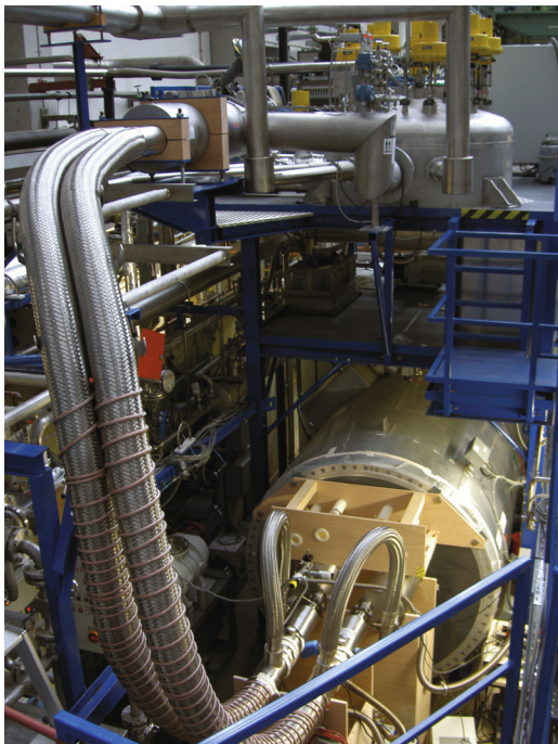
Fig. 1: Left: The new flexible TIMO-2 cryogenic transfer lines, equipped with heaters (for acceptance purposes). Right: Moisture condensation on top of the lines under cryogenic conditions inside due to inefficient insulation vacuum.
