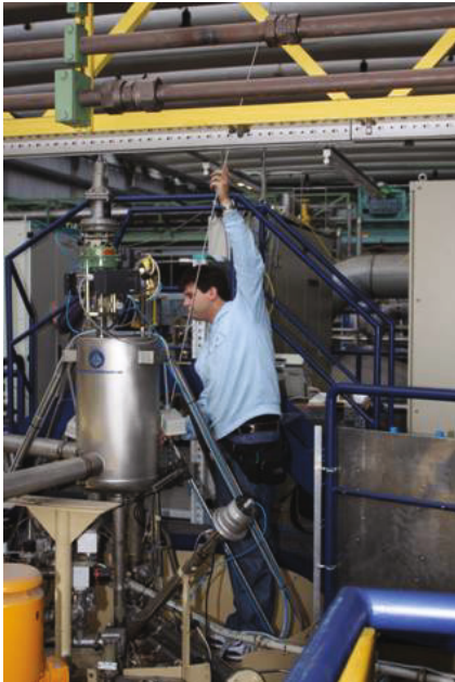
Fig. 4: Change of a temperature sensor for the 5,000 litre LHe vessel of the 300 W-refrigerator.
