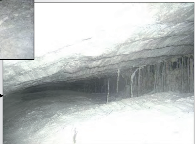
Open gaps below the roof at 700-m-level, photos taken at 04.12.2008
