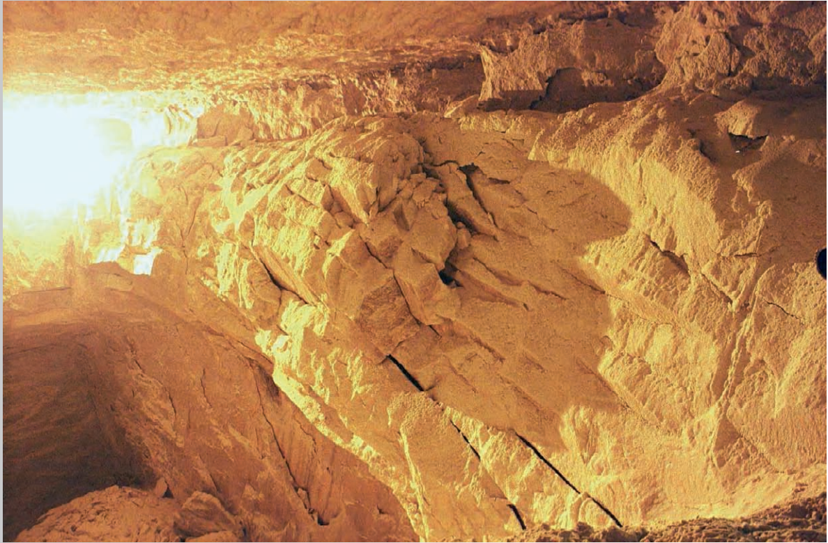
Broken stope between level 490 m and 511 m in pillar row 7, photo taken at 27.08.2003
