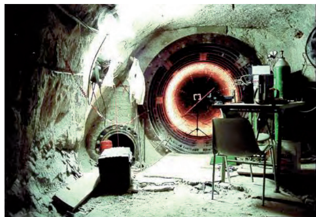
ALOHA 2: Bulkhead drift on the 700-m level
