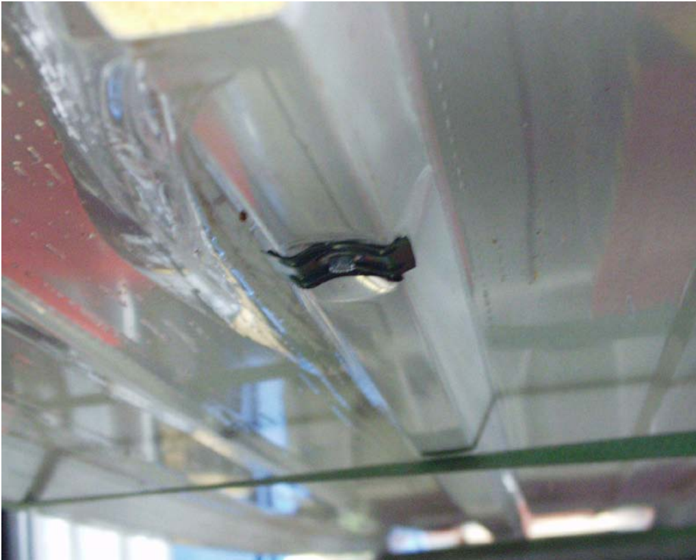
Fig. 16: Indentation of fastener, deformed saddle washer and web crippling
