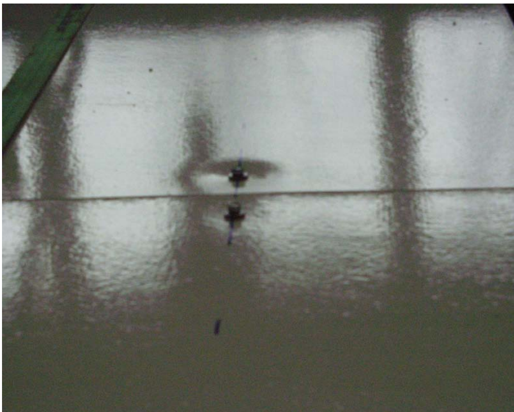
Fig. 8: Indentation of fasteners in the upper face
