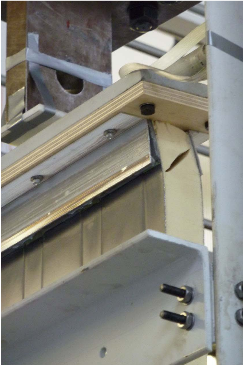
Fig. 14: Failure mode of test no. 05
