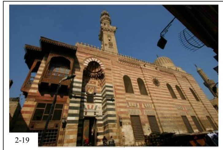
Figure 2-19: Recess bay includes the windows flanking the prayer niche and the bulls-eye in Madrasa of Sultan Barsbay
