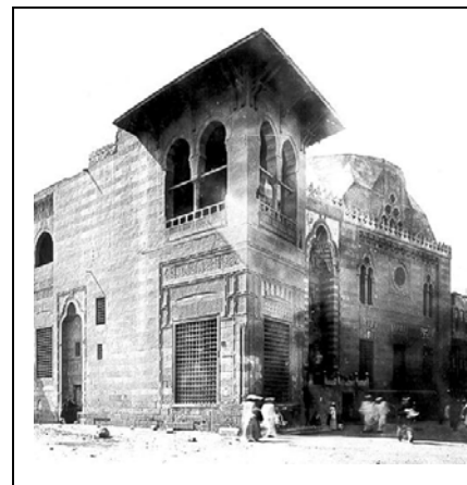
Figure 4-8: The sabil is beside the entrance in Madrasa of Sultan al-Ghuri
