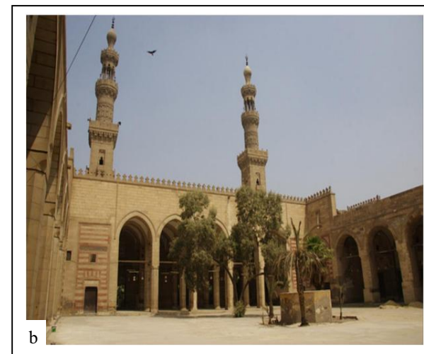
Figure 2-4: The spatial order of the centralized open courtyard model a- Madrasa of Sultan Hassan, b- Khanqah of Sultan Faraj Ibn Barquq
