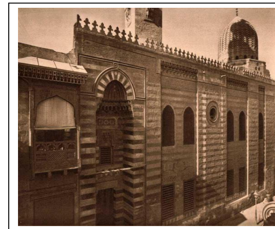
Figure 5-43: The main facade in Madrasa of Sultan Barsbay
