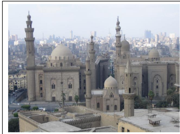
Figure 4-12: The mausoleum dome in Madrasa of Sultan Hassan
