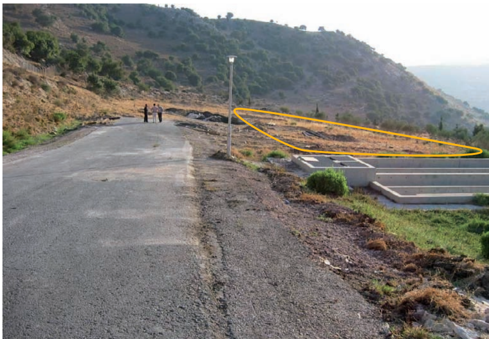
Figure 5.3 Topographical view of the selected site at Fuheis prior to the construction phase of the demonstration plant and irrigation fields
