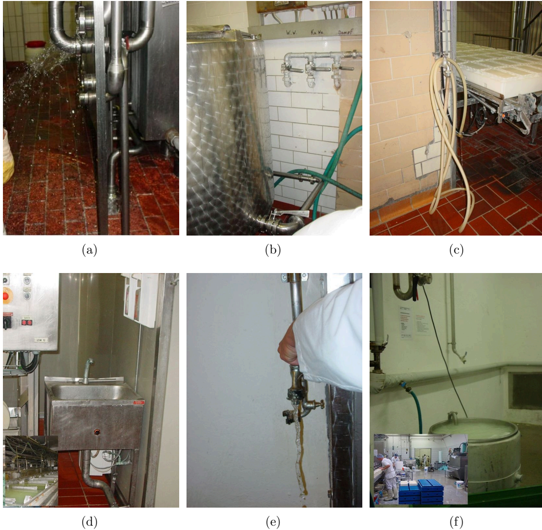
Figure 4.6.: Sampling points of German dairy company. (a) 1. Entry of public conditioned drinking water: reference, (b) 2. Lactic acid tank: water used to rinse the tank, (c) 3. Portioner: water used to rinse the portioner machinery, (d) 4. Hand washbasin: water used to wash hands in salting room, (e) 5. Maturation room: water used to clean the room, (f) 6. Feta packaging: water used to clean room and machinery.
