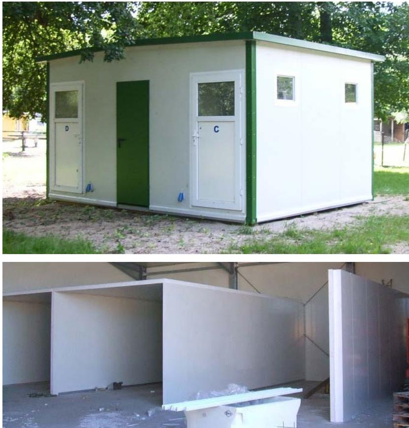
**Fig. 1.1: Buildings made of sandwich panels but without substructure**
