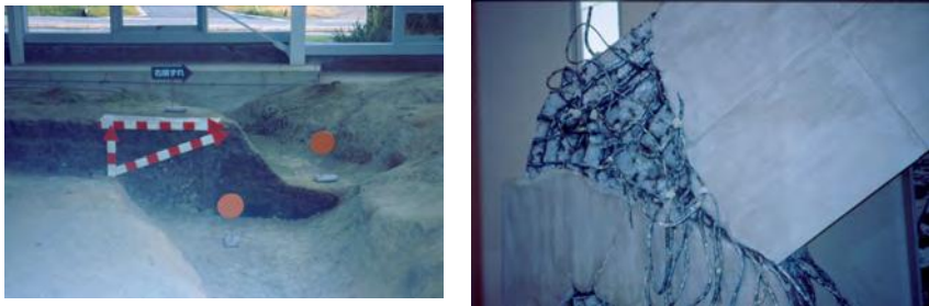
Fig. 18 Kobe earthquake. Relative displacements along the fault (left), plastic hinge in a column of a fly over (right)
