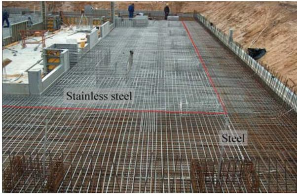
**Figure 4.5: Magnetic materials in the KATRIN hall.** This photograph shows the KATRIN main spectrometer hall when it was built. It is visible that in the central region of the hall stainless steel was used, whereas in the walls and in the floor close to the walls normal steel is embedded into the concrete.
