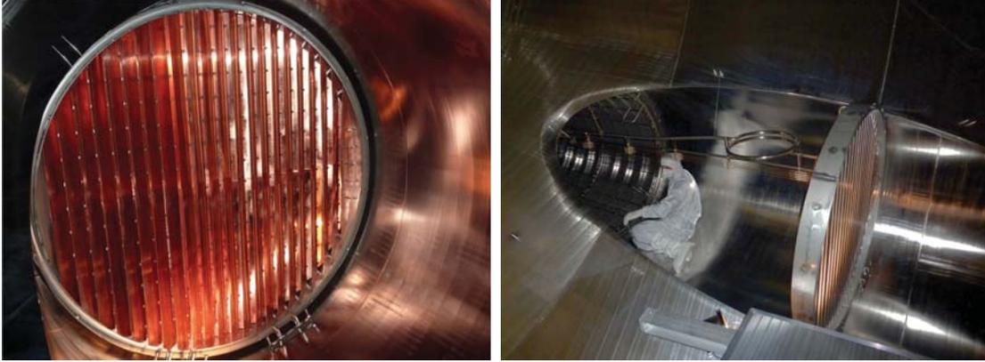
**Figure 6.19: Photograph of the cryo-baffle installation at the main spectrometer pump port.** Left: Photo from the front side. Face-on, there is no line of sight to the getter pumps installed in the pump ports. Right: The baffle, as seen from above, shows the cylindrical crate holding the NEG getter strips, as well as the cryogenic feed and return lines to cool the baffle to LN2 temperatures.
