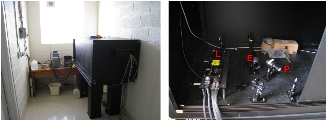
Figure 8.2: The Distant Laser Facility operated in the engineering phase until August 2010. In the left picture, the optical table and the flashlamp with the cooling system can be seen. On the wall on the left side are the circuits controlling the hatch on the roof. On the right picture, the optical components are shown. The laser (L) is directed through a beam expander (E). Afterwards, part of the light is picked off and sent to a pyroelectric probe (P). The rest of the light is diverted into the sky.
