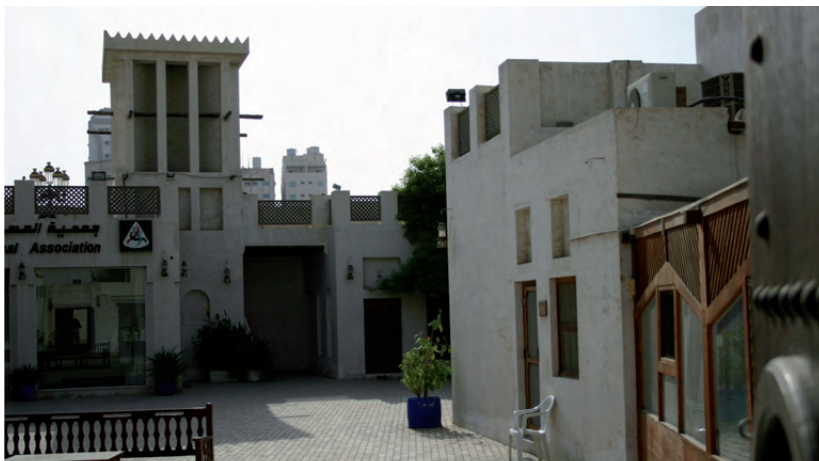
Figure 6: An example of a wind tower topping the left part of the building in old Sharjah (Source: author)
