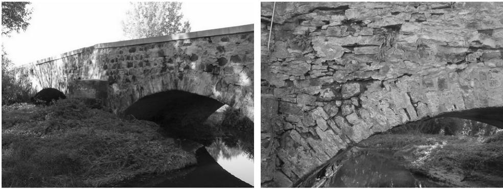
Fig. 4 Gyöngyöspata Bridge (left), Damaged, cracked spandrel wall (right)
