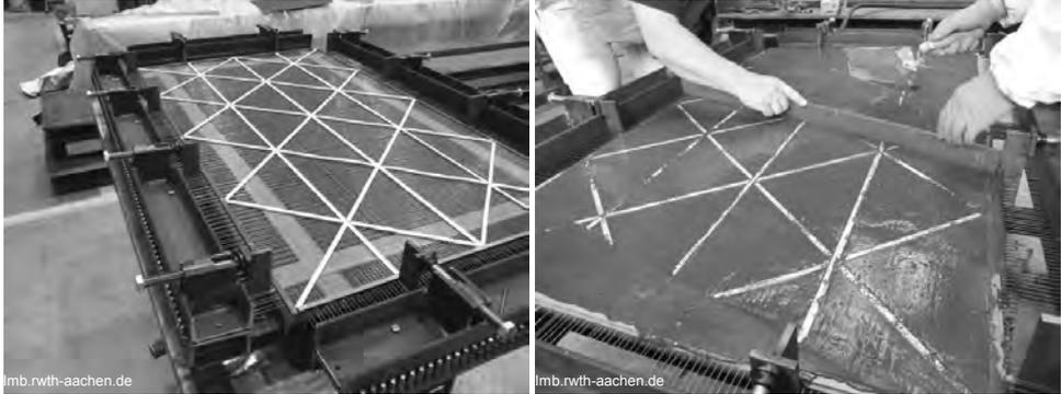
Fig. 2 (left) Reinforcement with spacers; (right) Placing of concrete
