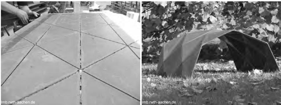
Fig. 3 (left) Concrete after hardening and removal of the spacers; (right) Completed structure after folding and filling the creases
