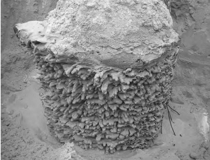
Fig. 1 The pit of a jet-grouting column (J. Bzówka [3])
