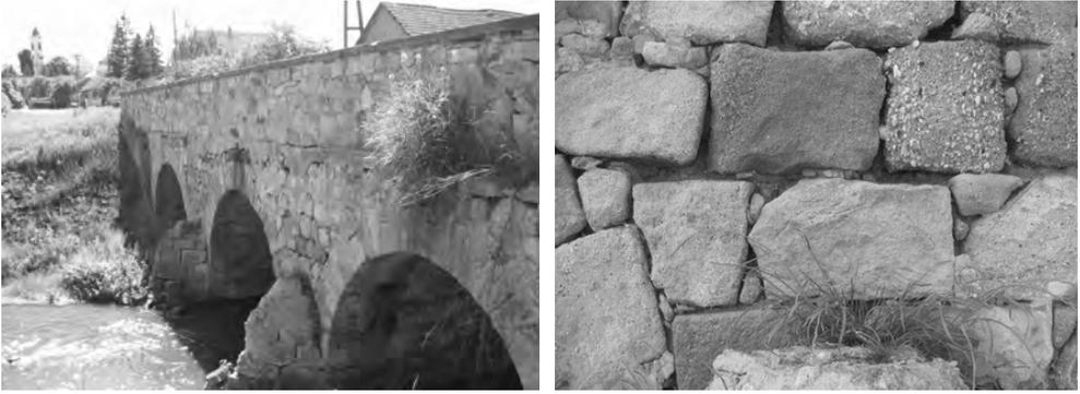
Fig. 2 Bridge over the Derék brook (left), Mortar loss on the bridge (right)
