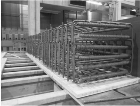
Fig. 3 Reinforcement edge beam (a)
