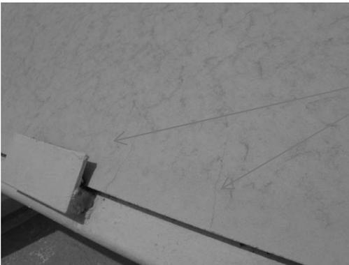
Radial cracks propagating from the edge of the panel due to the temperature elongation of the support structure.
