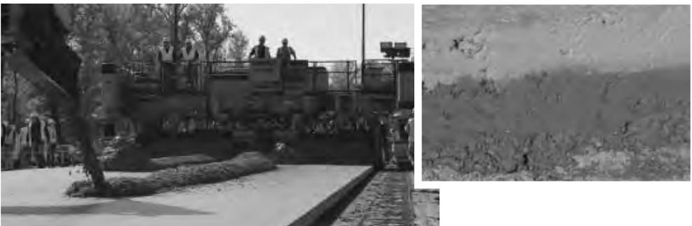
Fig. 4 Construction of a road with photocatalytic surface in St. Louis (left). The lower layer made of standard application concrete was experimentally covered by 5 cm of photocatalytic concrete (right). Reprinted from [9].
