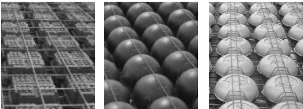
Fig. 1 Biaxial hollow core slabs: hollow cores in a box form (left), hollow cores with a spherical form (middle) and new hollow cores with a rotationally symmetric flattened form (right).
