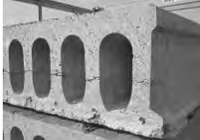
Fig. 1 Horizontal cracks in the webs above the strands of a HCS250 type hollow core slab.
