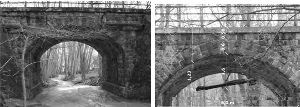
Fig. 1 Bridge over the Bükkös brook (left), Basic dimensions to the MEXE method (right)
