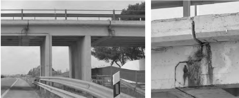
Fig. 1 Dapped-end beams in overpass of CV-500 road near Valencia, with accumulation of moisture
