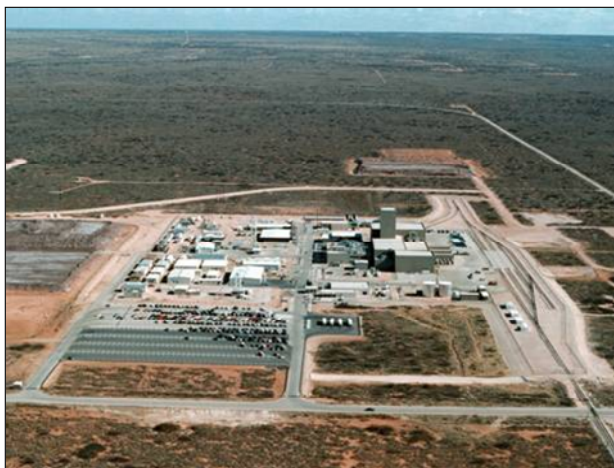
Fig. 1: Waste Isolation Pilot Plant (view of surface facilities) has operated for 12+ years as a repository for transuranic waste in a bedded salt formation
