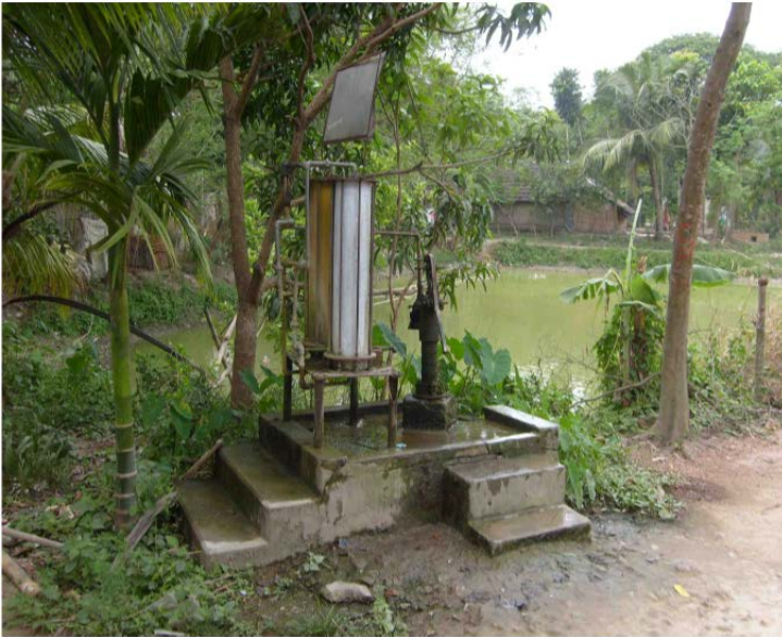
Figure 5.4: Picture of a public well installed in 2003 in the village Chakudanga, which is equipped with an As filter cartridge (well depth: 163 m). Surprisingly, the As concentration in filtered water was higher as compared to the raw water ( 77.4 compared to 101 \mu\text{g L}^{-1} ), strongly suggesting that the filter material needs to be replaced. This example demonstrates that current mitigation strategies (use of deep wells and filter systems) can be unreliable.
