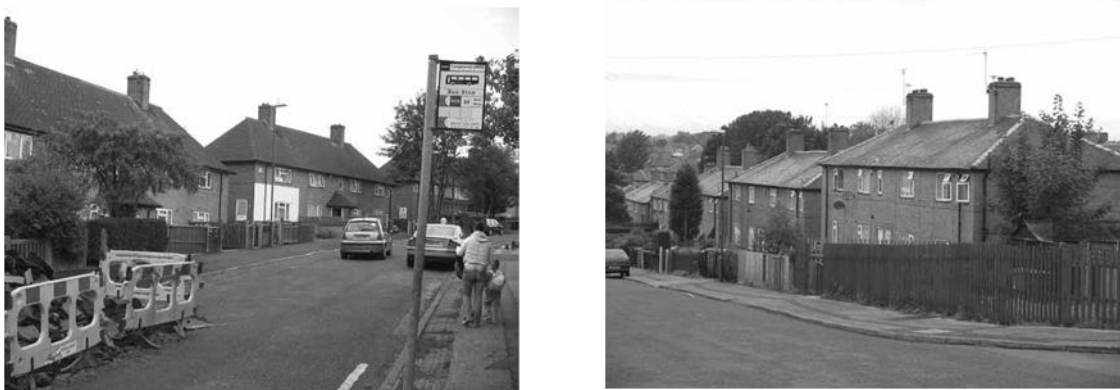
Figure 3-5: Photographs of houses surveyed (Allinson 2007), figure 10-2 (image courtesy D. Allinson)
