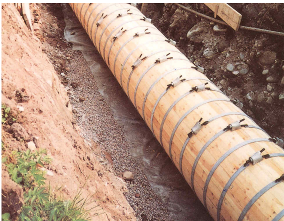
Fig. 2: Wood stave pipeline (a) in a ditch and (b) on bearings (Zwick GmbH, Canbar Inc.)
