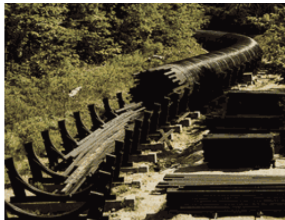
Fig. 2: Wood stave pipeline (a) in a ditch and (b) on bearings (Zwick GmbH, Canbar Inc.)
