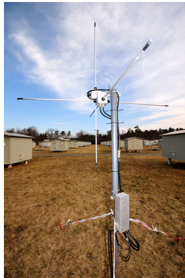
Figure 3.0.1: The three crossed dipoles of a LOPES-3D antenna station
